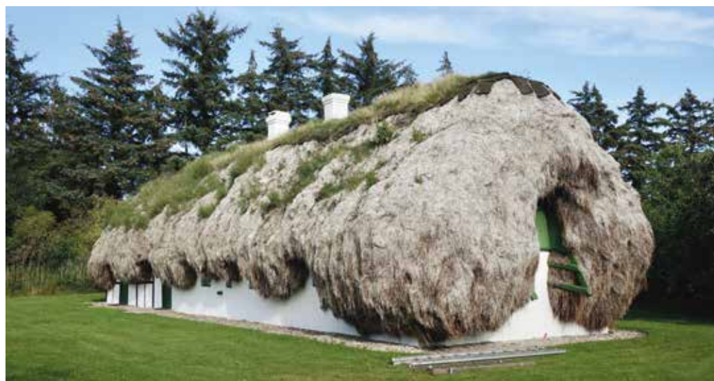
House in Laesoe, Denmark with a traditional seaweed roof. This particularly durable type of construction is found along the Danish coasts
